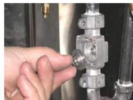
7. Remove and replace the spring/magnet assembly.
