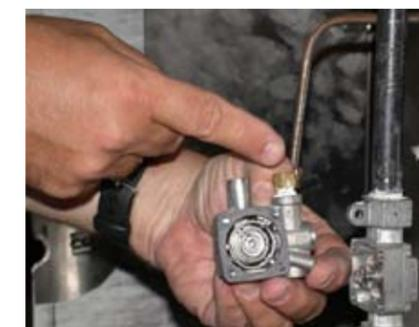
6. Remove brass adaptor attached to the safety head and install on the new head.
