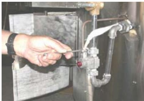
1. Using a  $\frac{3}{8}$ " wrench, remove the thermocouple from the control.
