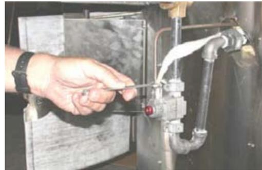
2. Using a  $\frac{3}{8}$ " wrench, insure the thermocouple is snug in the body of the safety control. A good rule is giving a  $\frac{1}{8}$  turn after finger tightening. **DO NOT OVERTIGHTEN** as it will damage the control.
