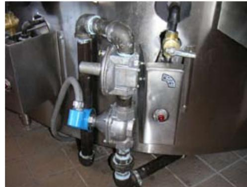
2. We recommend a 2" gas supply line. Minimum line size is 1½". Large MBR units will not perform as designed if an insufficient gas line cannot provide adequate supply volume.
