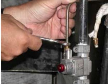
11. Carefully thread the brass fitting from the pilot gas line into the body and tighten using a 7/16" wrench.
