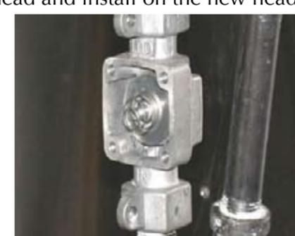
8. New spring/magnet assembly installed.
