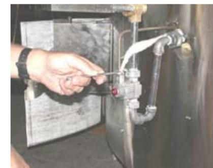
2. Using a 3/8" wrench, remove the brass thermocouple fitting from the safety control.
