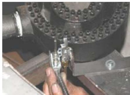
2. Using a  $\frac{7}{16}$ " wrench, remove and replace the thermocouple from the pilot burner bracket. When installing the new thermocouple, be sure to thread the adjusting nut up to the top of its travel.
