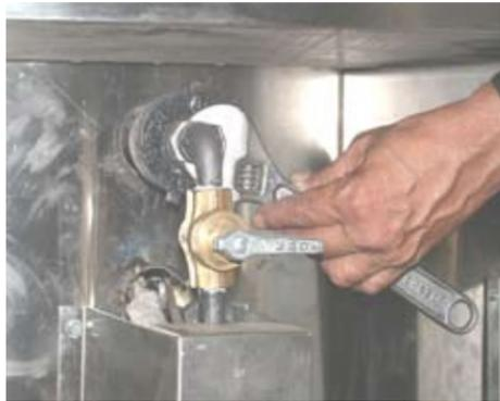
**The gas burner orifices are fixed, but the amount of air can be adjusted..**
